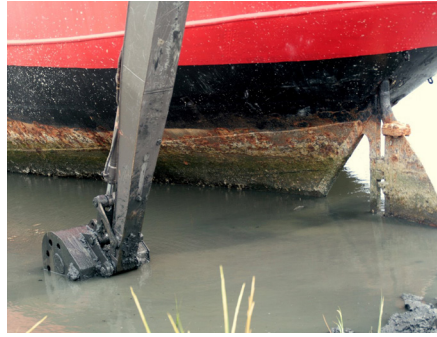
Mechanically dredging the mud out from around the ship in the slip.
