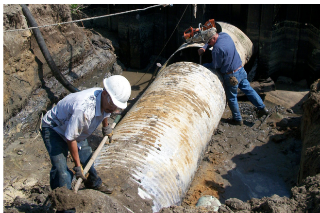
Replacing the end of the 48" pipe.
