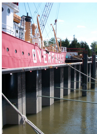
Left: View from the bow, note the tieback rods and mooring piles. Right: Line handlers being put aboard with forklift.
