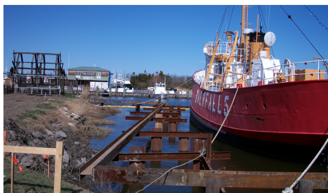
Port side template used to guide the sheet pile.
