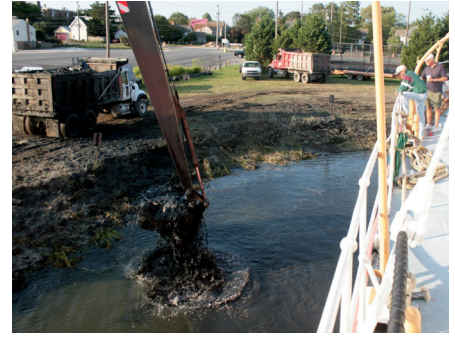
The mud goes into the truck for transport to the USACE spoil site on the other side of the canal.
