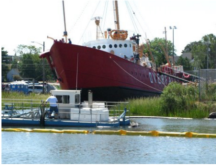
Hydraulic dredging the area from the slip to the channel in the canal.
