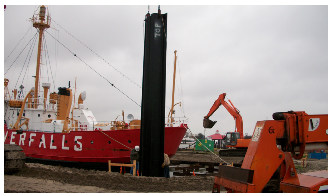
Driving the first piece of sheet pile in a heavy rain.
