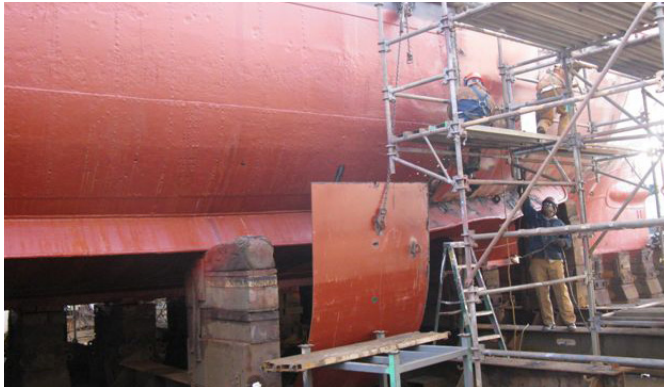
New hull plate being lifted into place
