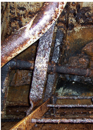
Left: Fuel tank prior to cleaning and painting.
