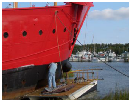
Top: Before and after painting the hull red (black bottom) before and after. Bottom: Painting the hull from platforms and aerial lift.
